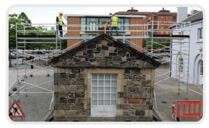
Spandeck links 2 towers for chimney maintenance in Belfast.
