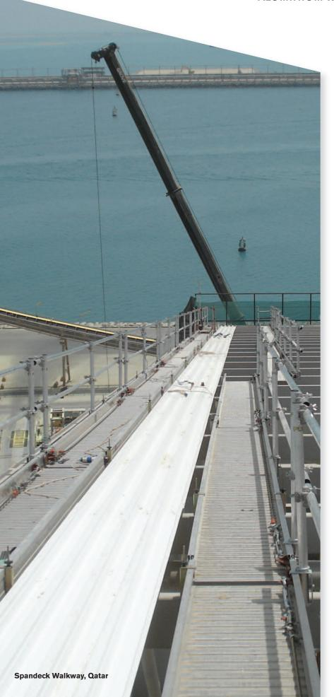
The Instant UpRight Spandeck system is a lightweight walkway, bridging and staging system. This system provides a safe, simple and cost effective solution for even the most bespoke of applications. Lightweight for easy handling, yet durable for the most arduous of applications.
