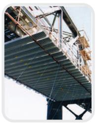
Linked Spandecks provide a platform for under bridge refurbishment.
