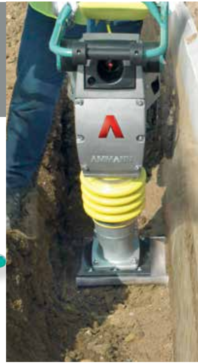
340 mm asymmetric: compaction work in trenches protected by shuttering systems without inclining the rammer during operation
